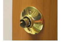
Slide on the extension until the clip fits into the slot.
