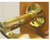
NOTE: If the handle does not stay on, use a 7/64" bit to drill a larger hole into the handle so that the set screw has a better grip when you back it out.
