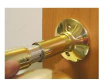
Slide on the door handle. The pin hole should line up with the set screw on the shaft. If it doesn't, loosen the set screw in **Step 5**. Go back to **Step 4**. This time, don't pull the extension out so far.
