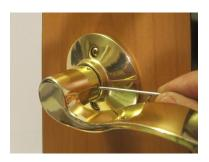
Insert a thin rod through the hole at the base of the door handle. Push to release the handle
