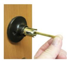
Pull out the thumb turn lock and slip the lock extension onto the shaft.
