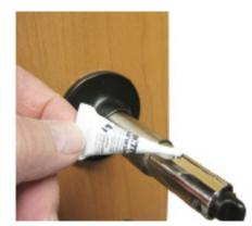
Dry fit the door handle before applying Loctite adhesive in the top and bottom grooves.
