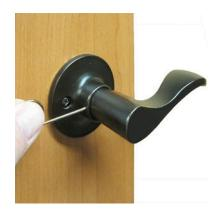
Use a pin to release the door handle. Remove the handle.
