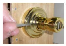
Insert a thin rod through the hole at the base of the handle. Push to release the handle.
