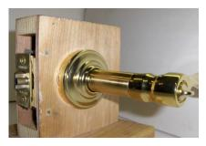
Push on the outer extension until it snaps into place. Turn it back and forth to seat it into the slot. Hold the extension straight and tighten the set screw on the opposite side.
