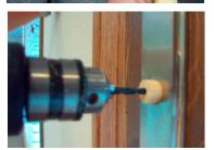
Replace the escutcheon plate on the door. Insert the nylon centering piece and drill a 3/16-inch pilot hole completely through the door, keeping the drill level and straight.
