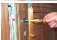
Now attach the interior escutcheon plate onto the long spindle. If the spindle resists, loosen the set screw until the spindle goes in. Then tighten the set screw after Step 12.
