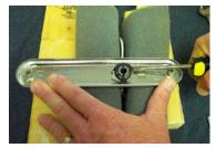
Remove the escutcheon plate from the door and save the screws. Remove the press nut from the back of the escutcheon plate using the tip
