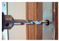
Remove the wooden centering piece. With a 7/16-inch bit, drill a hole just past halfway through the door. Now finish drilling the 7/16-inch hole from the other side of the door.
