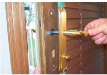
Now attach the interior escutcheon plate onto the long spindle. If the spindle resists, loosen the set screw until the spindle goes in. Then tighten the set screw after Step 9.
