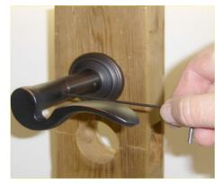
Replace the door handle. Line up the hole in the handle over the extension set screw. Turn the screw counterclockwise until the handle is secure.
