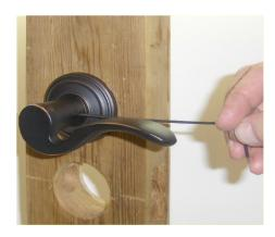
Because the set screw is reverse threaded, turn it counter-clockwise to loosen it. Remove the handle.
