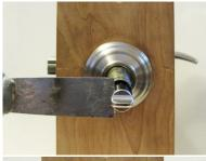
Insert a putty knife between the thumb-turn cap and the plastic base. Push the putty knife handle toward the door. Do not pull up because this might break the cap. If one putty knife doesn't pop the cap loose, use two putty knives from opposite sides. Always push the putty knife handles toward the door.
