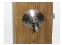
Replace the door handle. Line up the hole in the handle over the extension set screw. Turn the screw counterclockwise until tight. If the handle does not slide on completely, see if the set screw is catching.
