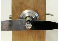
Insert the thumb turn extension until it snaps into place. Tap on it with a hammer if necessary.
