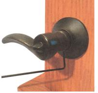
Use an Allen wrench to loosen the set screw
