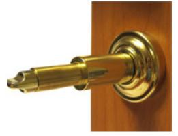
Insert the thumb turn lock into the extension.
